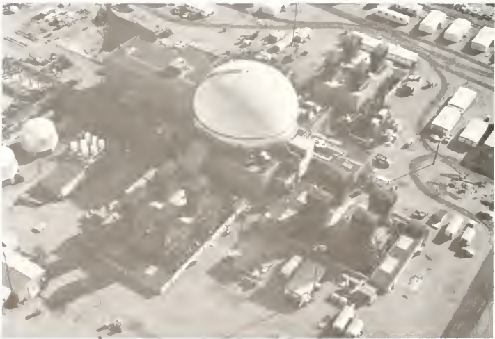
View of the fast flux test facility on the Department of Energy's Hanford site, 7 miles north of Richland, Wash. The FFTF will test breeder reactor fuels and materials. The Science Committee authorized the project, at a construction cost of $647 million.
